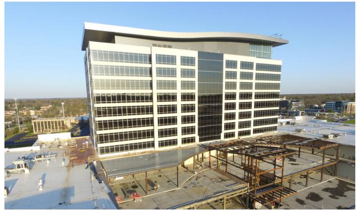
3D laser scanning measured 1.54 million square feet of retail, office and parking garage space with millimeter accuracy.
