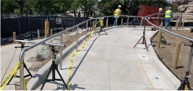
Precise as-built data ensured the railing system would fit properly when delivered and installed.
