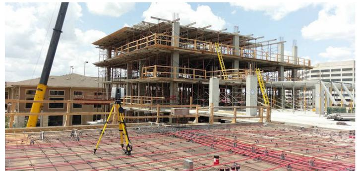
TruePoint 3D laser scanned an eight-story apartment complex over an 8-month period to capture the existing site conditions prior to the slab being poured.
